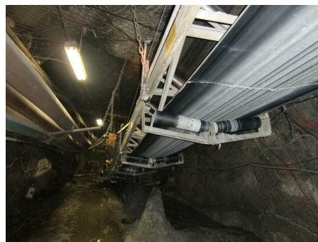
COAL MINING CONVEYER BELT WATER-MIST PROTECTION
